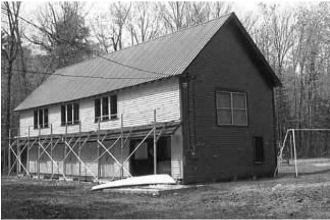
Structural work in process at Shop
