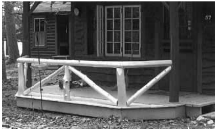
New railing ready to be painted on the Camp Mother's Cabin
