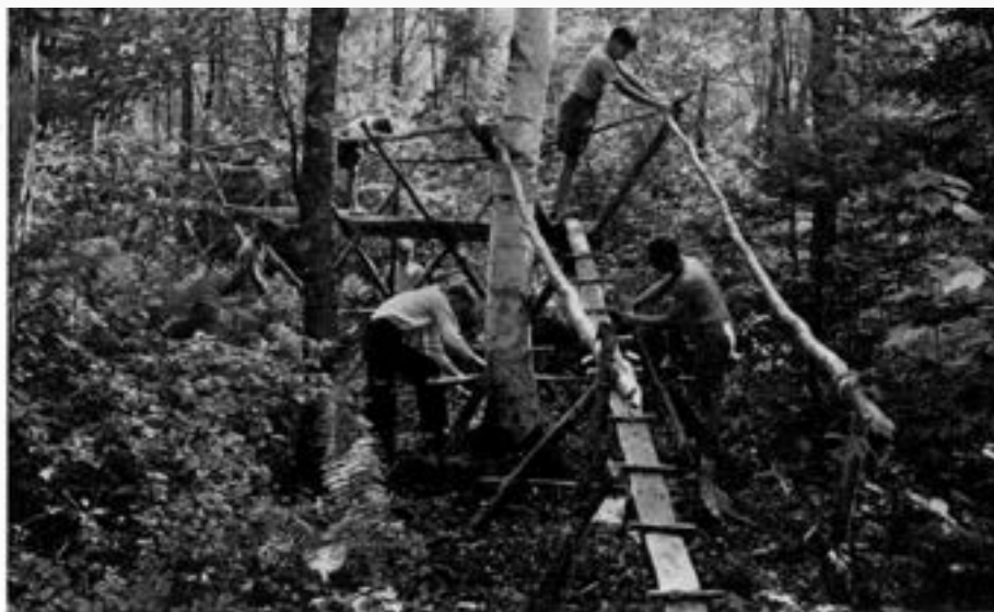
The Monkey Bridge Nears Completion
